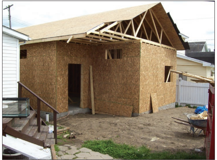
The amazing before and after photo of the exact same area at the GGGH as the foundation goes in, top, and then new structure!
